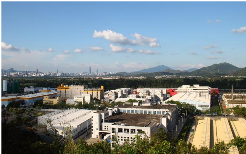
LCA-07 Yuen Long Industrial Estate
